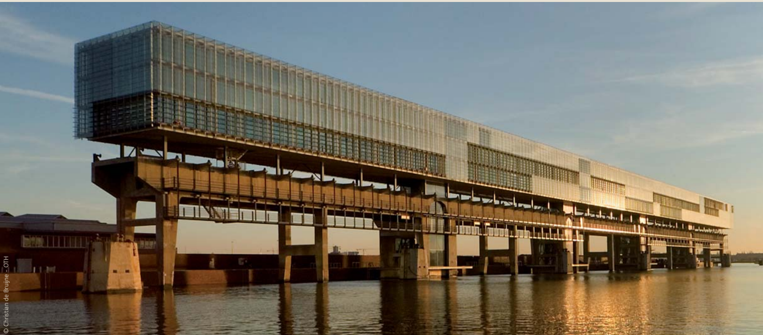
Kranspoor: re-utilisation of a old concrete crane for a new innovative steel framed office building - MIPIM green building Award
