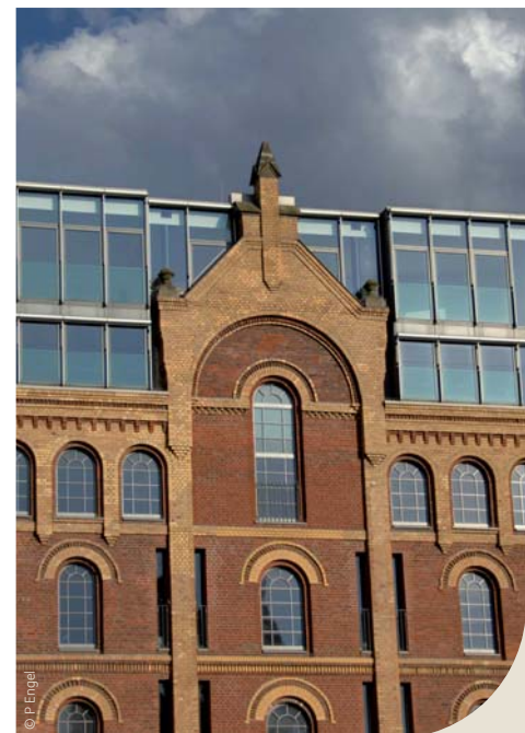
Dusseldorf: surelevation of an historical brick building
